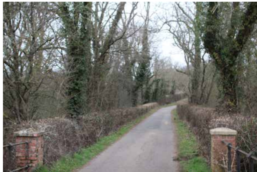
E. Bridge over River Kird - view north
