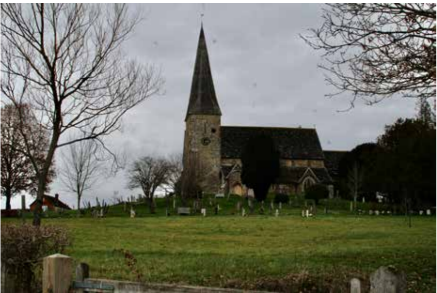
D. Billingham Road - view north
